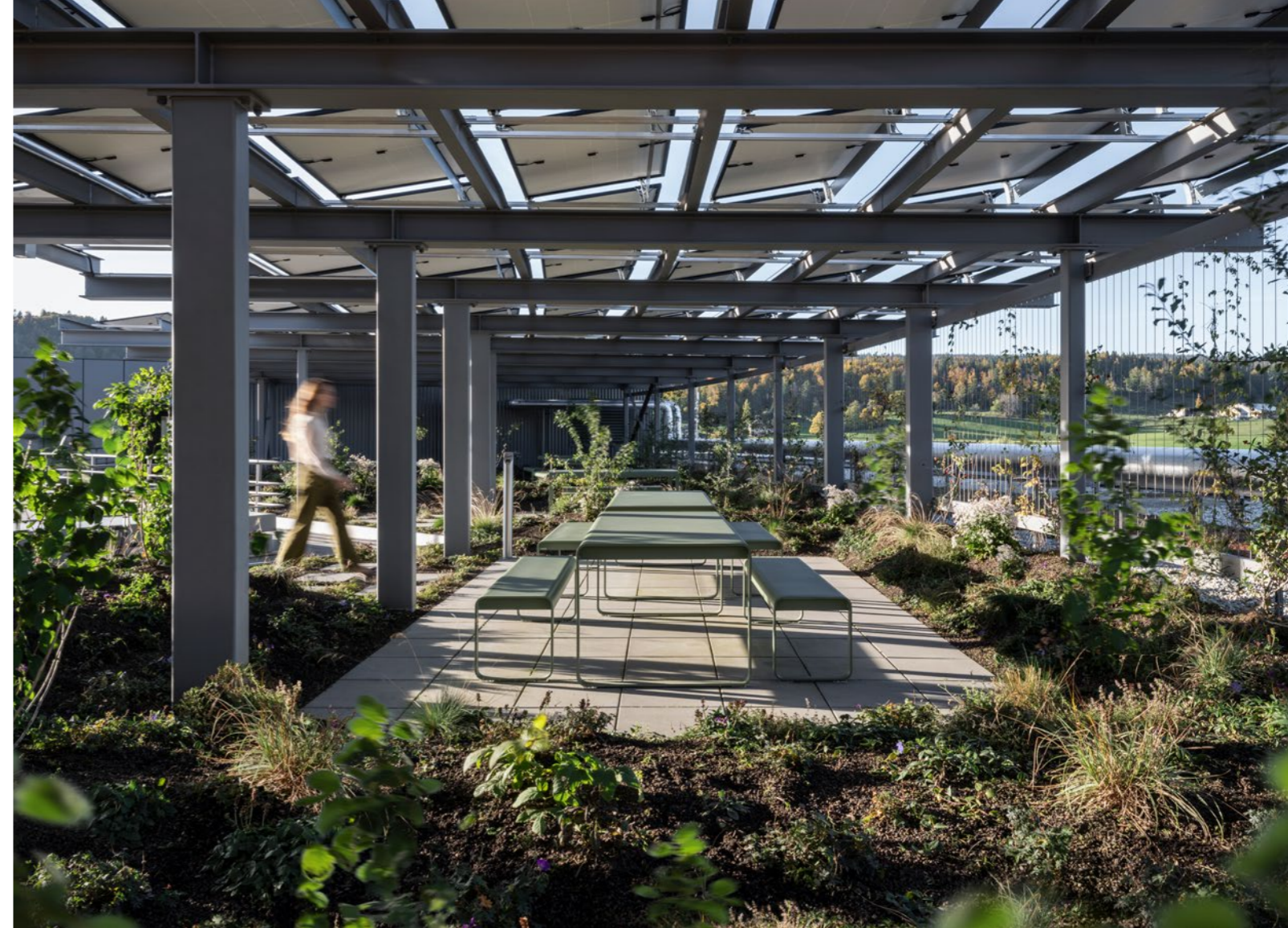
Solar panels on the rooftop of the Manufacture du Brassus - Le Brassus, Switzerland
